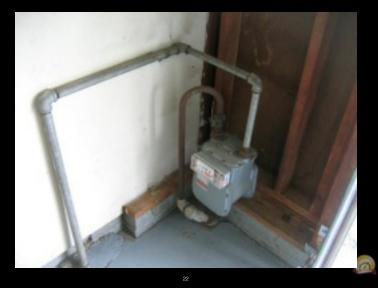
rust peeling paint physical/mechanical damage ice/frost inadequate access possible gas leak tilting poor installation shut-off valve
