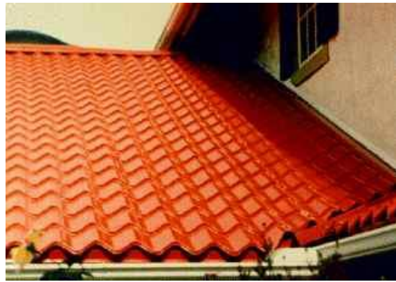
Above: This is also a metal roof -- in this case, designed to look like Spanish tile.
