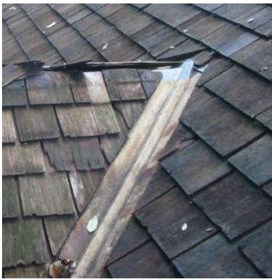
Above: a metal open valley on a poor-condition wood shingle roof
