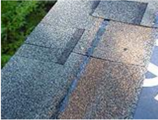
Here, you can see the side-lap between overlapping shingles.
