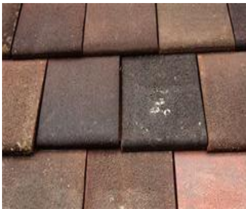
At left: a flat clay tile roof
