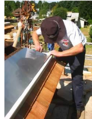
Above: a Yankee gutter being installed together with its metal flashing. The earliest Yankee gutters had no flashing at all.
