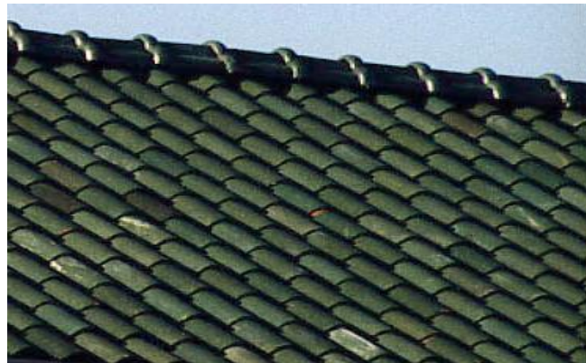
At right: a glazed clay tile roof
