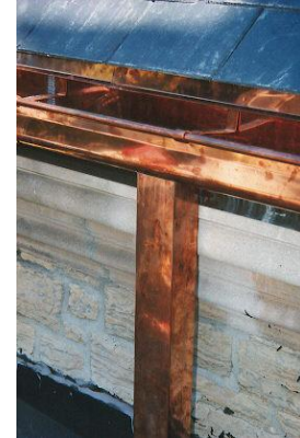
Above: copper guttering in new construction; note the copper drip edge.
