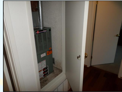
5.1 Item 4(Picture) Closet in hall
