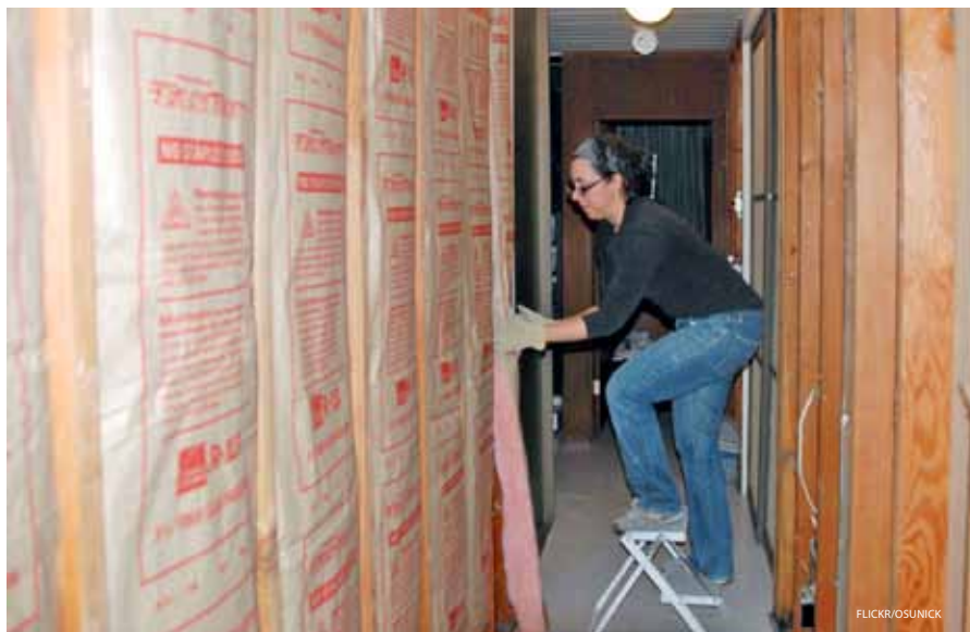
Installing high efficiency insulation.
