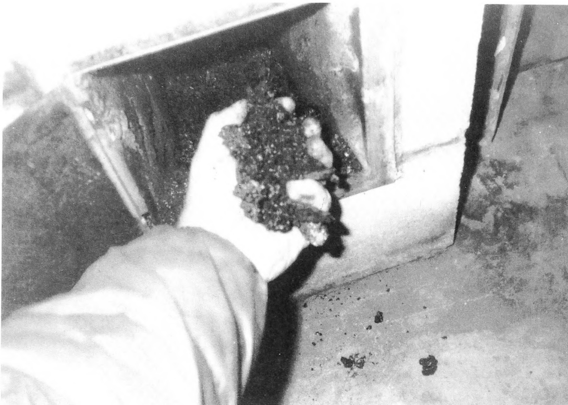
Fig. 1-27. Never allow creosote to build up to the extent that you can take handfuls out, as seen in this photograph.
