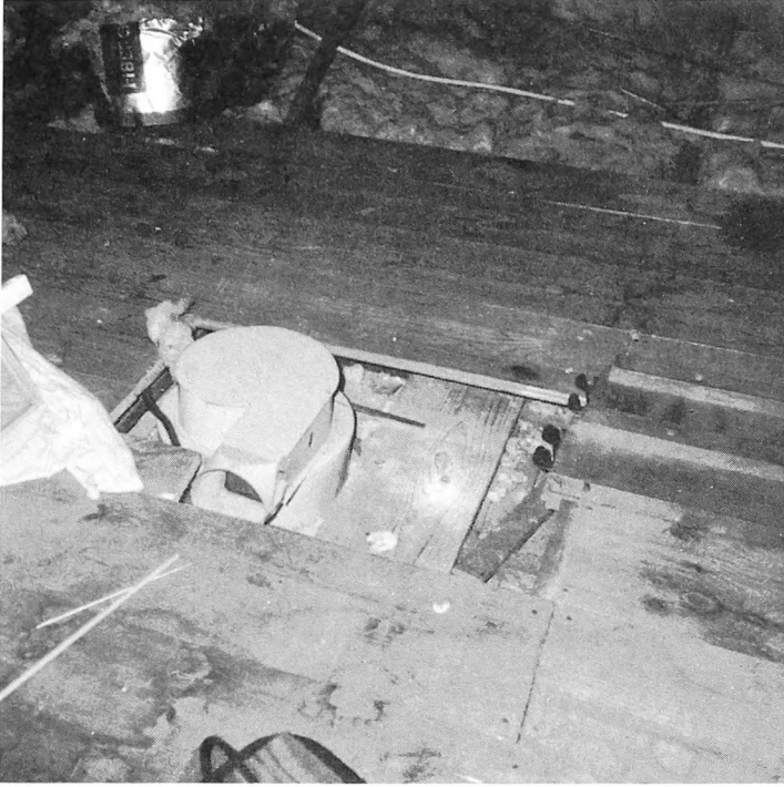
Fig. 3-13. If you are presently venting bathroom moisture to your attic or crawl spaces, you greatly increase your chances of condensation.
