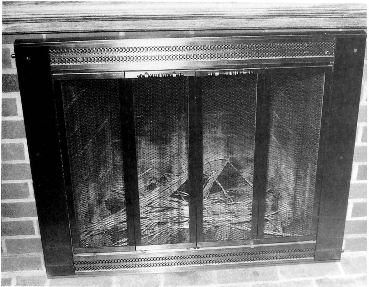
Fig. 6-8. Fireplace enclosures need to be caulked and sealed to keep out unwanted drafts and to avoid heat losses from the building.
