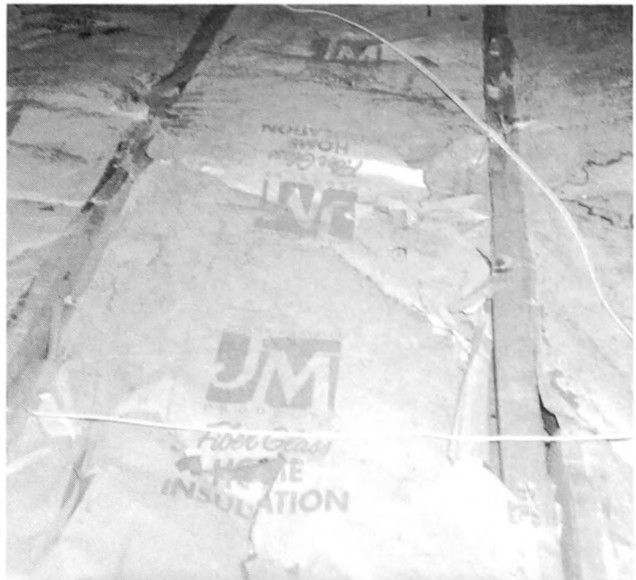
Fig. 3-7. Vapor barriers in exterior walls are crucial to a building's health. Incorrectly installed vapor barriers will do more harm than good, producing condensation that will damage both insulation and framing.
