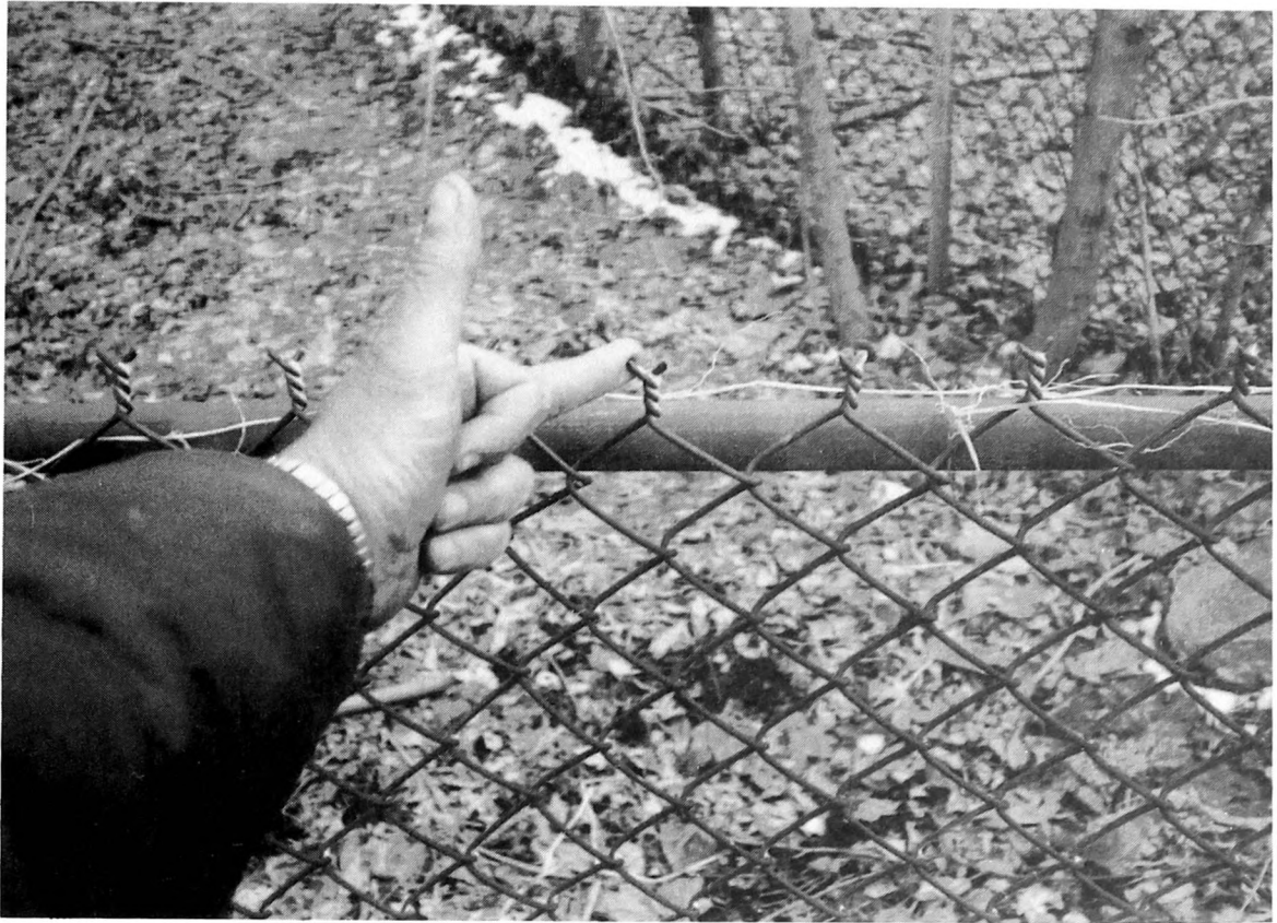
Fig. 1-16. Maintain fences on an annual basis. Make sure there are no potential hazards, such as exposed metal barbs.
