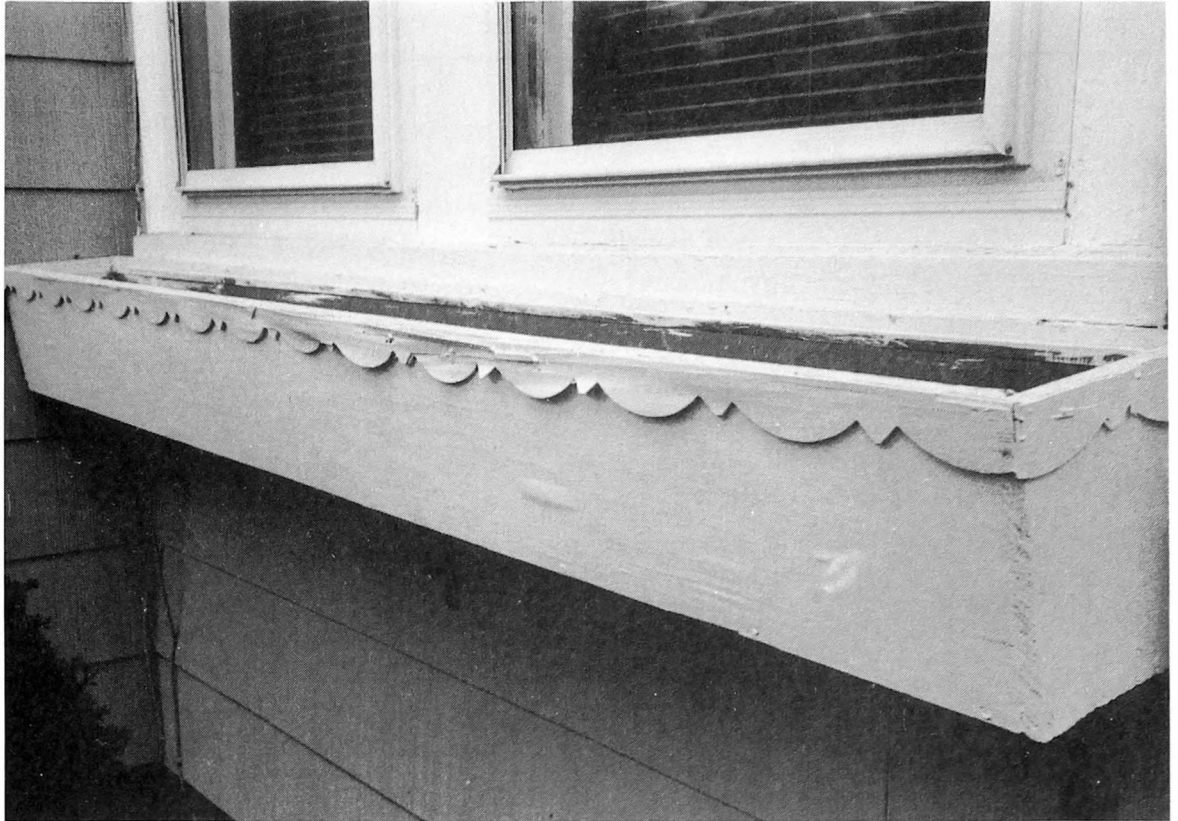
Fig. 5-12. Do not place wood planter boxes adjacent to the building. Even with treated wood, some moisture will be drawn to the building siding resulting in decay.
