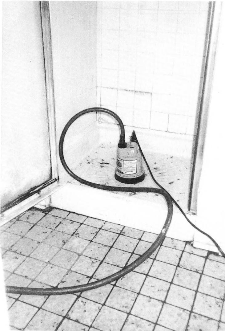
Fig. 7-32. A sump pump is relatively inexpensive and should be part of every building's equipment. All buildings can be subject to flooding under the right conditions.
