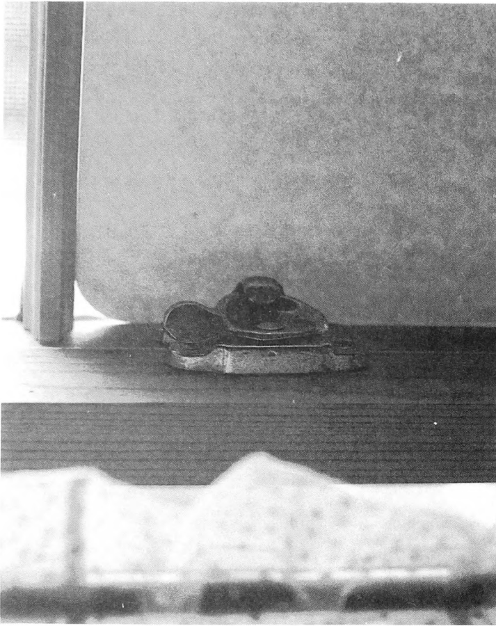
Fig. 6-15. Window hardware such as the clamshell latch provide a tight seal between the upper and lower windows. If you have windows without such locking devices, be sure to add the chore of installing them to your maintenance list.
