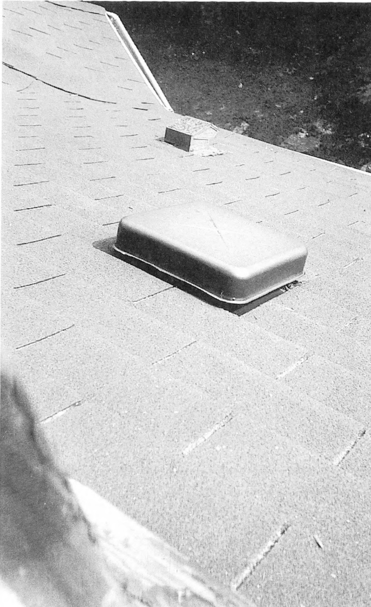
Fig. 6-13. A roof-mounted vent. Usually if these units are used alone without any corresponding airflow from opposite directions, their effectiveness is questionable.
