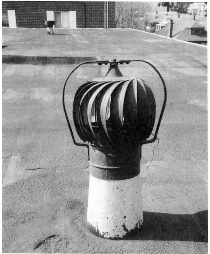
Fig. 6-11. A roof-mounted turbine vent. Vents that require wind movement or electrical means to vent out air are probably not the most efficient or effective. Natural air convection has proven, when used in combinations, to be the most effective and cost efficient.
