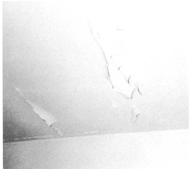
Fig. 4-4. On poorly pitched roofs, such as shed roofs, ice dams and ice damage will result under the right conditions.
