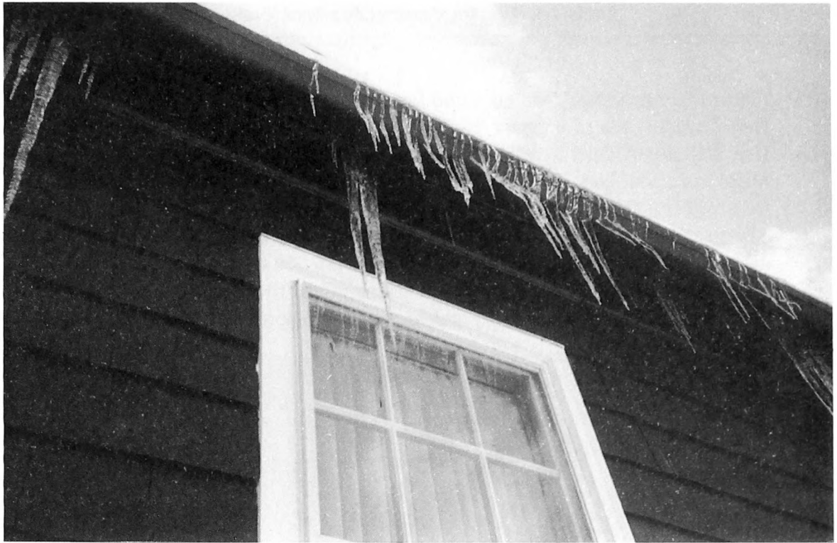
Fig. 4-4. On poorly pitched roofs, such as shed roofs, ice dams and ice damage will result under the right conditions.
