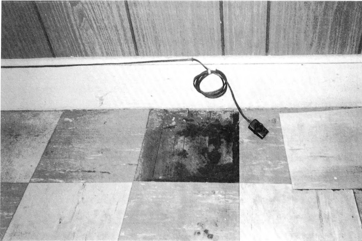
Fig. 7-20. Avoid using makeshift wiring such as lamp cord outlets. If you need additional circuits, have an electrician install safe wiring and outlets to meet your demands.
