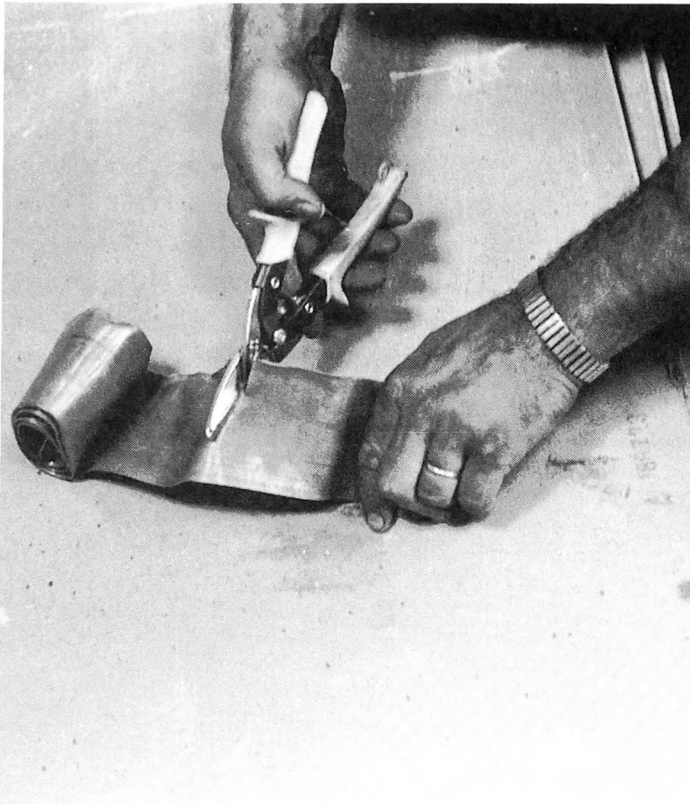
Fig. 4-8. Lead flashing can be cut to size and shape with metal snips.
