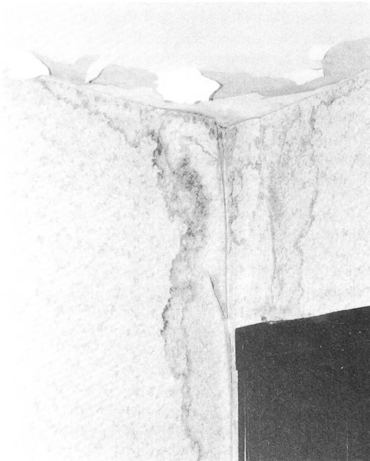
Fig. 8-1. Peeling paint in any building, but particularly older buildings, could signal lead paint hazard. Be sure to correct the source of the problem and then get rid of the peeling paint.
