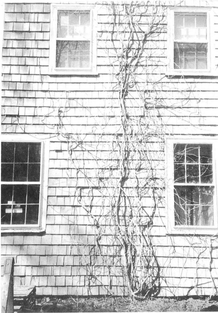
Fig. 1-17. Overgrown vegetation such as shrubs, plantings, trees, or ivy will result in decay and possible wood-boring insect activity. Keep all plantings under control.
