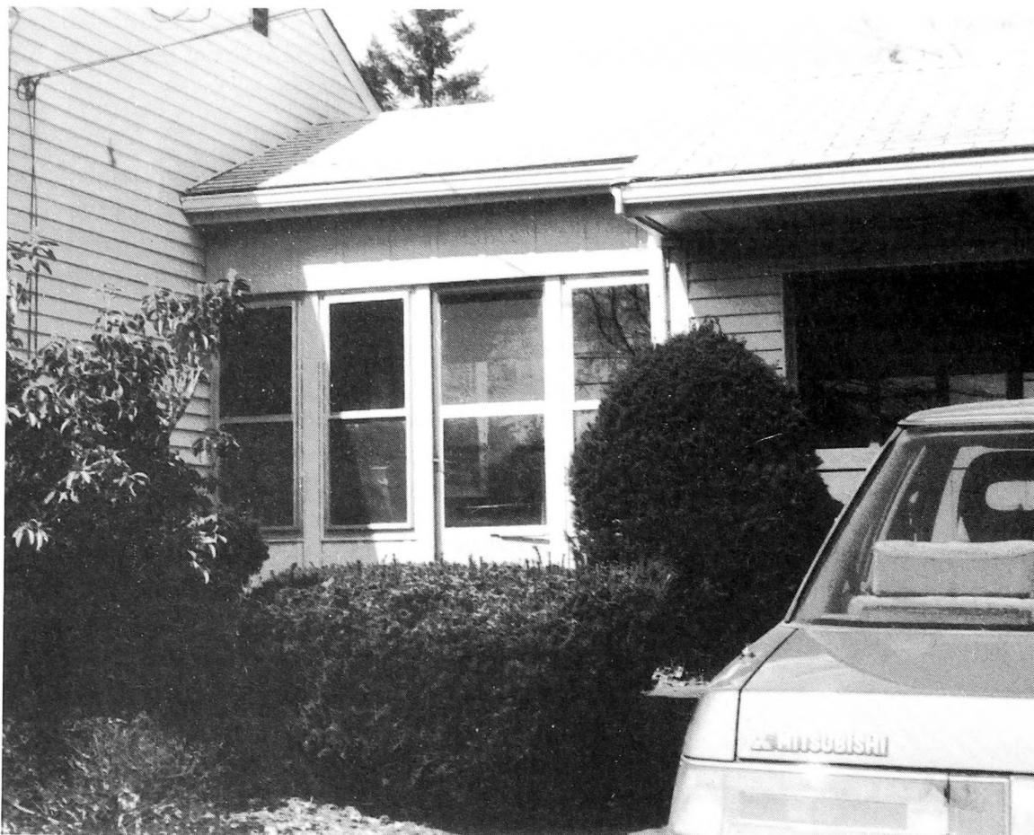
Fig. 5-11. Keep all of your plantings under control and several feet away from foundation areas as well as wood siding and trim areas.
