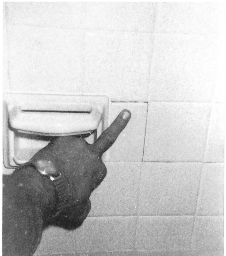
Fig. 1-26. Maintain joints in tile walls and floor areas by grouting and caulking periodically.
