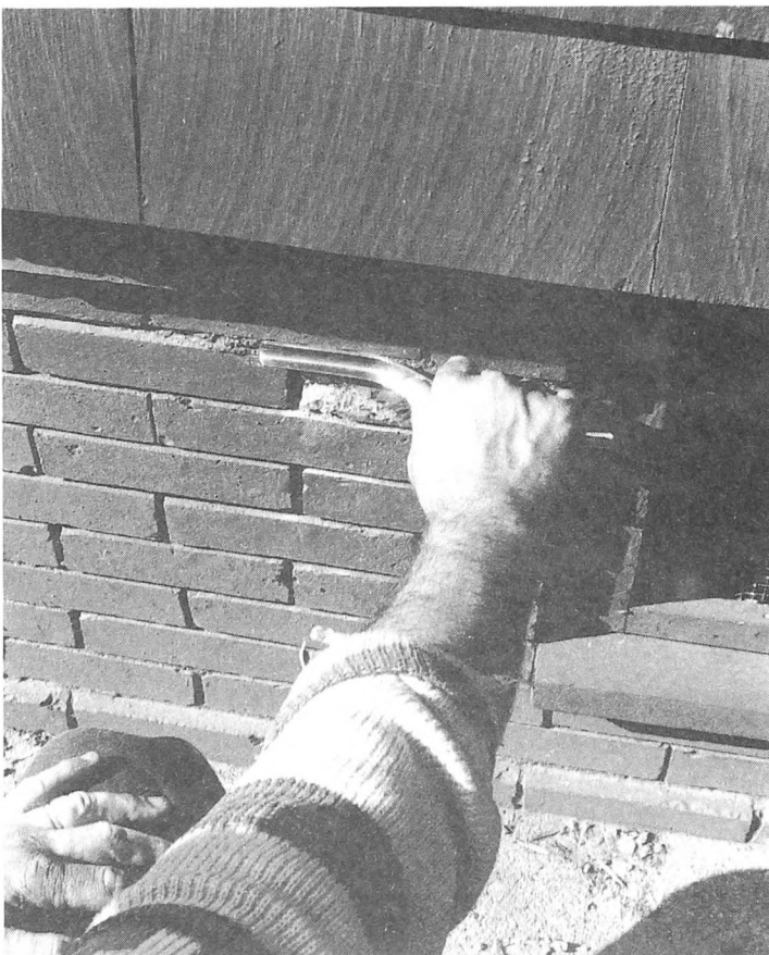
Fig. 2-13. Pack plenty of new mortar into the open joints. When you think that you can't apply any more, try forcing some more in.
