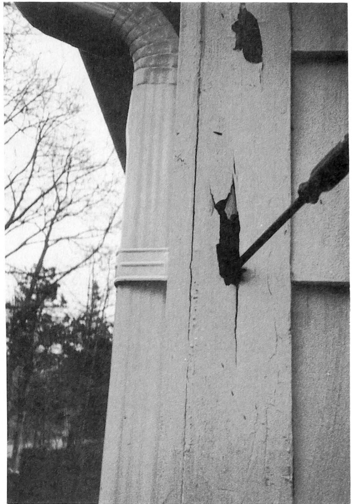
Fig. 5-16. Use a tool such as a screwdriver to probe suspect areas during your quest for termites. If you find hollowed out wood, you have had these unwanted guests, and they might still be lurking about.
