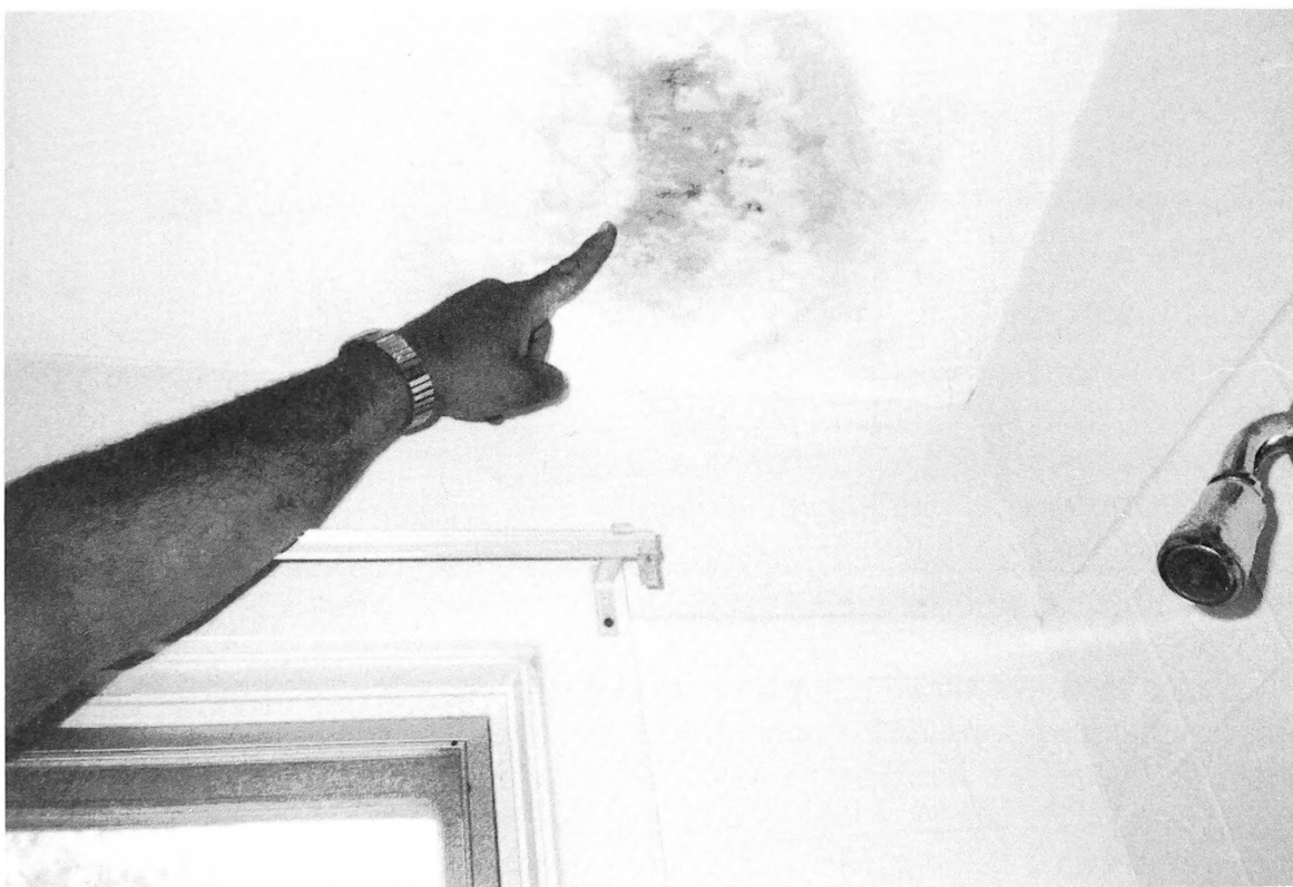
Fig. 3-27. The results of trapped moisture in a bathroom. This mildew growth will, if left unattended, cause serious damage to the ceilings and walls in this bathroom.
