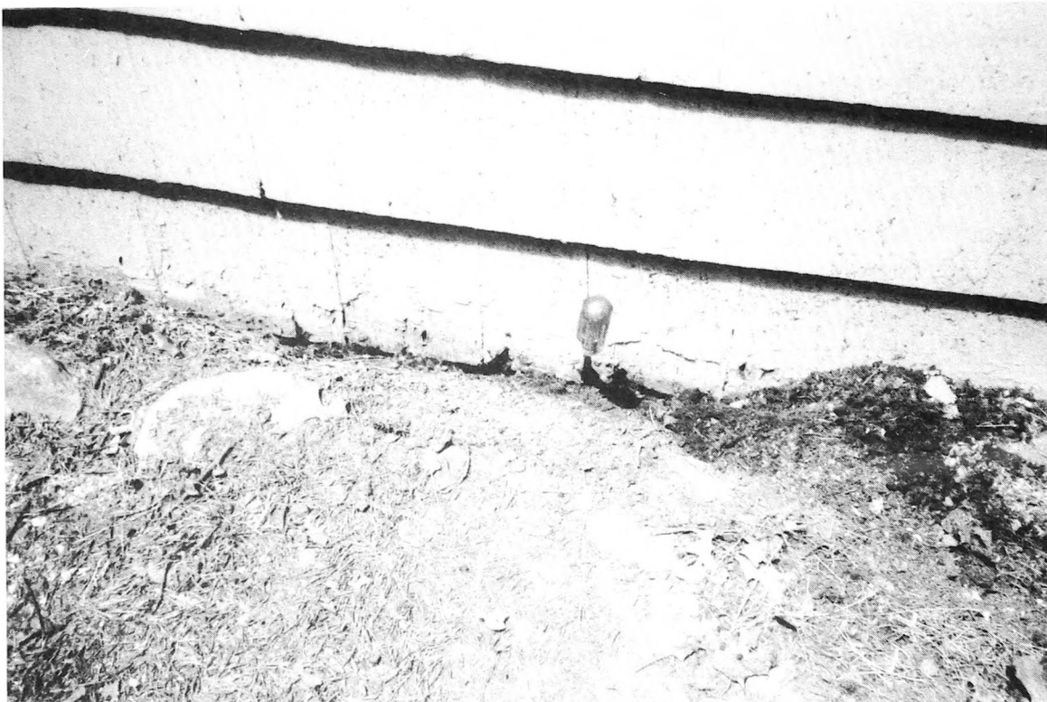
Fig. 1-12. Anytime that you have untreated wood in direct contact with the soil, you are tempting fate. Both decay and wood-boring insects will cause damage to such wood members.
