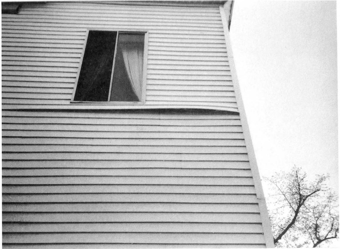
Fig. 3-11. Vinyl and metal sidings tend to hold moisture between them and the building framing. The end result usually is major decay and deterioration to the building. Additional ventilation is required for such buildings.
