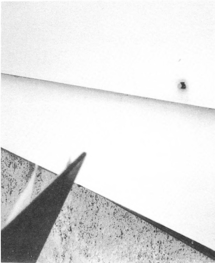
Fig. 5-8. Using incorrect types of nails that will rust can cause staining and eventual deterioration in siding and trim areas. The photograph shows the beginning of decay at the rusting nailhead.
