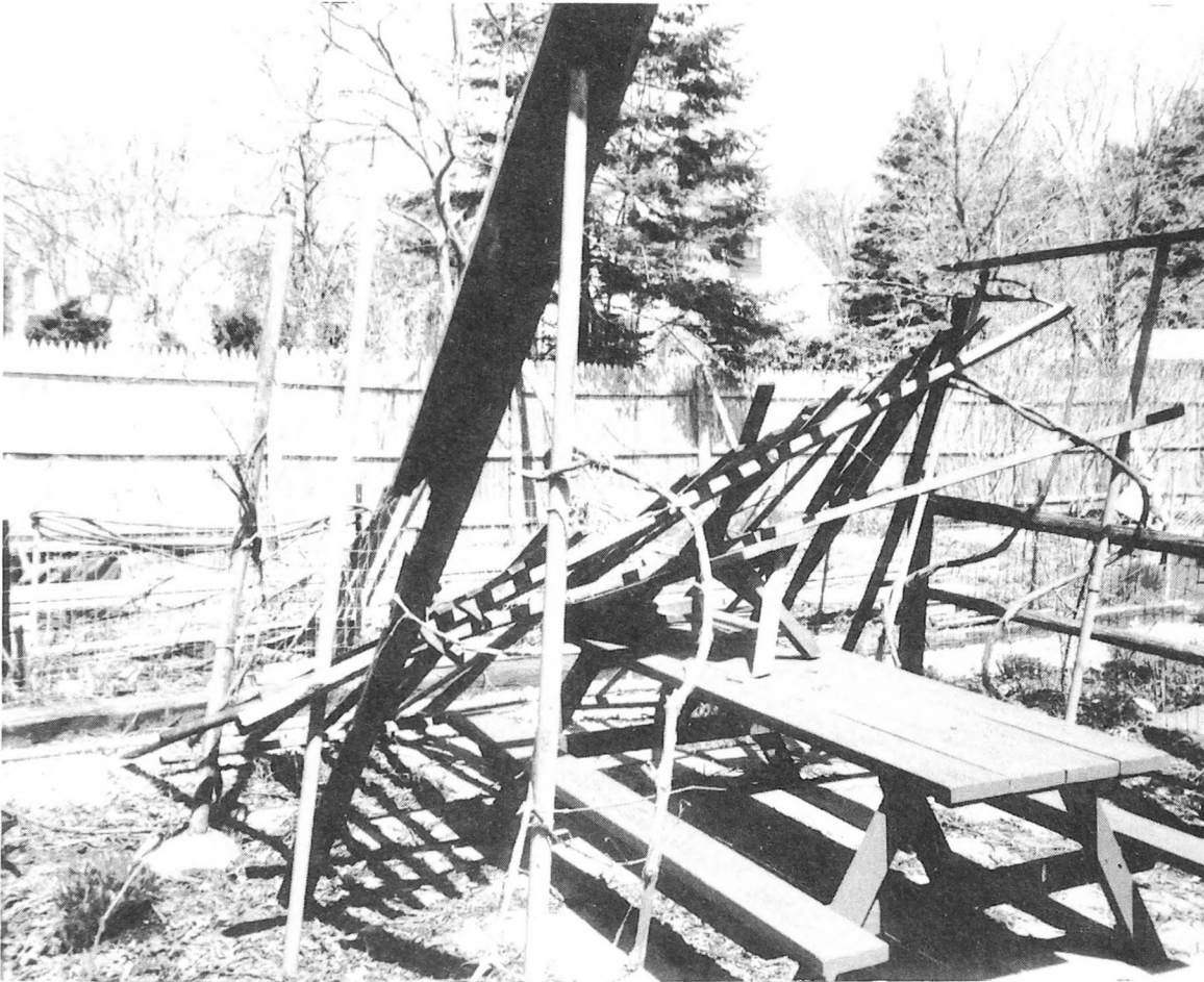
Fig. 5-9. Never use second-hand lumber or wood that is not pressure-treated for outdoor projects. Saving a few dollars cost this owner dearly in the loss of a grape arbor.
