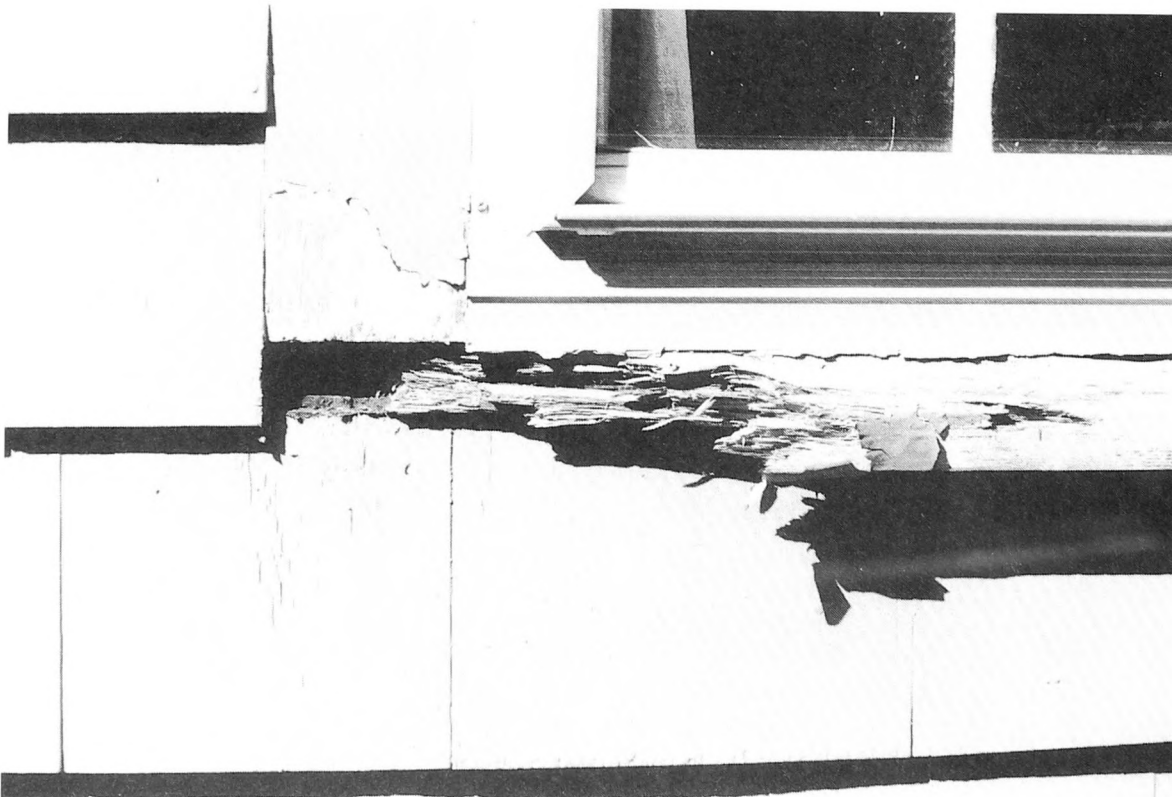
Fig. 4-30. Damaged and decaying wood trim can sometimes be the entry point for water penetrations.
