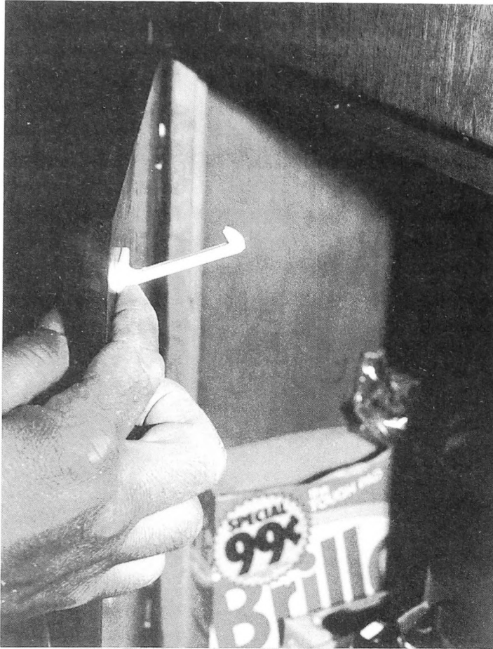
Fig. 8-20. Safety latches on cabinet doors prevent children from getting at dangerous substances.
