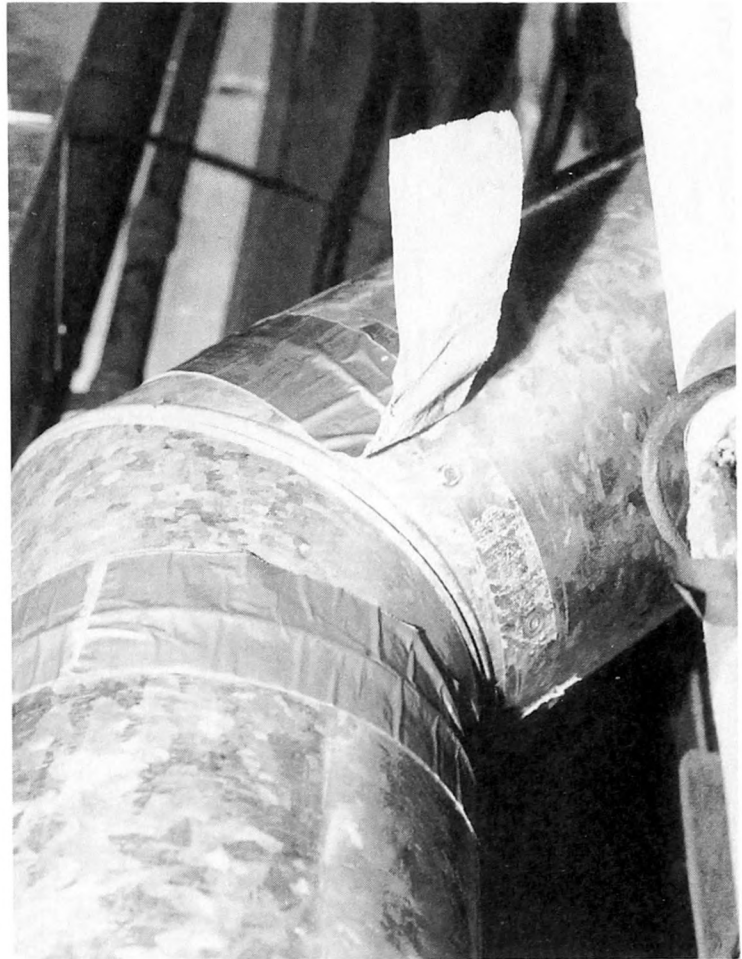
Fig. 7-11. Be sure that all heat duct joints are properly sealed with duct tape to avoid heat losses in basement or crawl-space areas.
