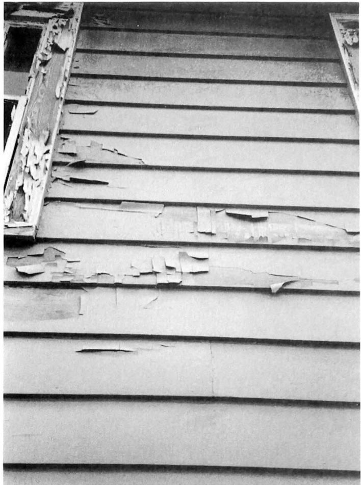
Fig. 1-10. Failure to provide sufficient ventilation in your building will result in moisture related problems.
